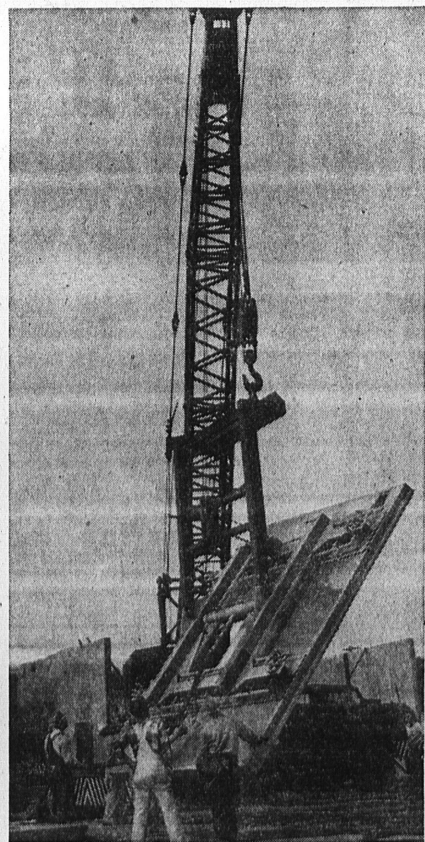
UP SHE GOES . . . A huge plate with vacuum grids pick up a wall section from the concrete slab which will later be a floor for another classroom.—Herald Photo.
