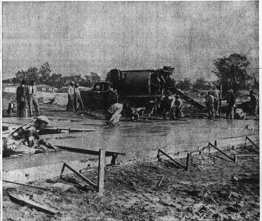
POURING THE WALLS . . . A huge load of concrete is being poured into the wall sections which have been formed on the site of the new Madrona Elementary School. After it had
