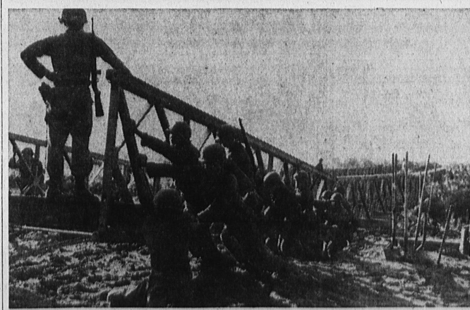
BIG PUSH... Soldiers in Torrance's 578th Engineer Battalion push multi-toned Bailey bridge across Japanese canal and into place during 40th Infantry Division field maneuvers on Japan's Honshu Island. The outfit constructed bridge recently while on three-day bivouac. Man at extreme left is a sergeant—no doubt! (U. S. Army photo).
