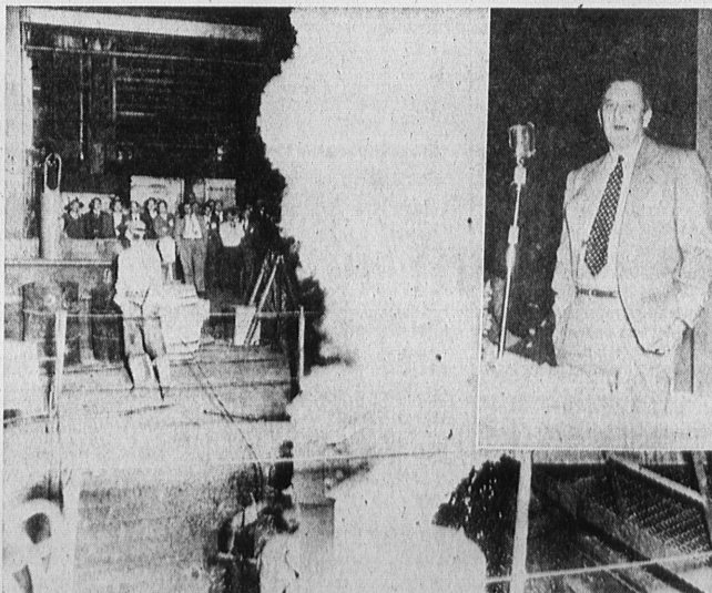
HOT STUFF... Half a hundred members of Southland management clubs watch as the giant electric steel furnace is emptied into a ladle before being taken to the various waiting molds at the National Supply Company's plant here. The clubs were visiting National Supply last Friday. Inset is George C. Ford. (Herald photo.)
