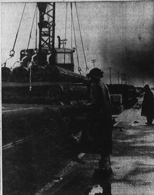
OVERSEAS CARGO ... Part of 300,000 feet of welded steel pipe is hoisted aboard ship at the Long Beach Harbor, destined for Israel. The pipe, manufactured by the Cal-Metal Corporation, a relative newcomer to the local industrial scene, will be used by the new nation for irrigation purposes. Pipe was nested to conserve shipping space.
