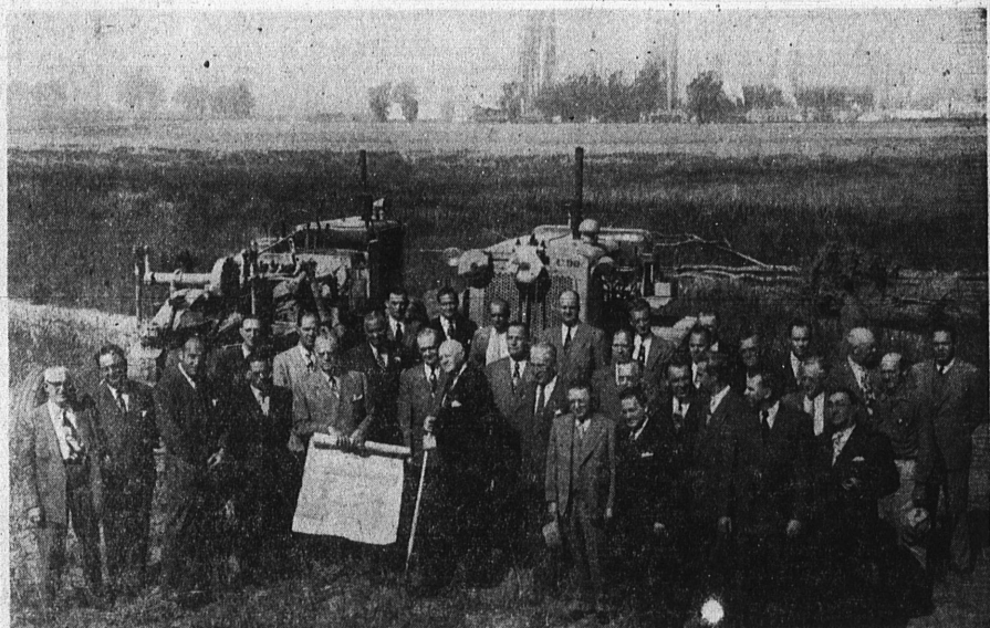
CONSTRUCTION STARTS... While civic leaders and neighboring factory executives beam approval, Torrance Chamber of Commerce President Charles Ver Jones (holding map) locates the spot for Louis F. Theurer, divisional director of the Pitts-
