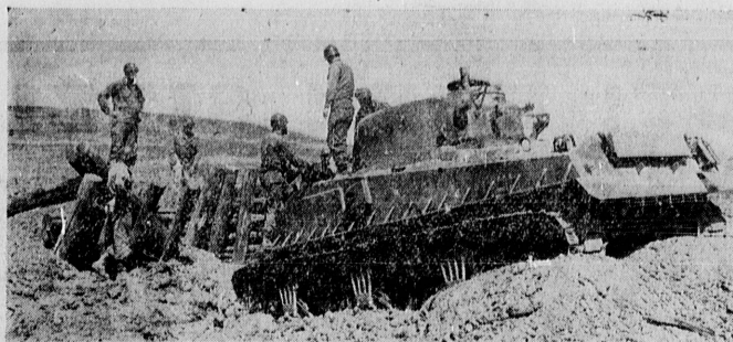
OUR ENGINEERS STOP 'EM —A 40th Infantry Division tank tries without success to break thru a tank trap constructed by the Torrance-Lomita 578th Engineer (Combat) Battalion. Hopelessly stalled during maneuvers at the Division's first postwar encampment at Camp San Luis Obispo last week, the crew is shown surveying the situation. Standing, left, is 1st/Sgt. Frank Savage, and immediately below him Sgt. J. Mitchell. Beyond Sgt. Savage is Lt. E. J. Hellmer, Company commander, and at right, standing on tank, is Capt. W. W. Ohlschlager. Tank driver is not a member of local battalion.
