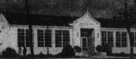
NEW CATHOLIC SCHOOL FOR TORRANCE . . . Pictured above is the architects drawing of the proposed Catholic School of the Nativity, to be constructed at Acacia Ave. and Carson St. on property recently acquired. A convent for teachers also is planned on a Cota St. site opposite the Catholic Church of the Nativity.
