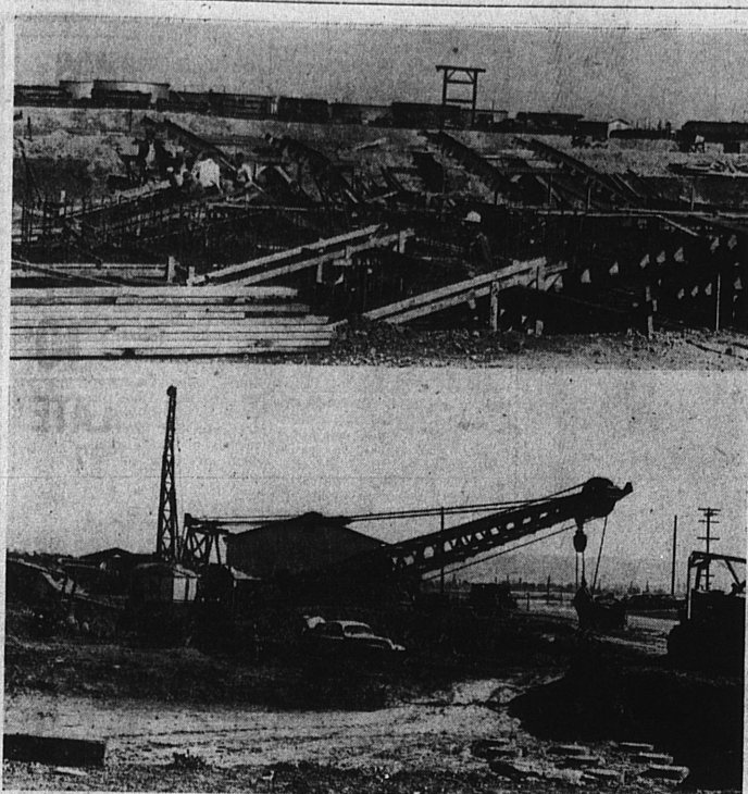
TORRANCE REFINERY BEING EXPANDED . . . General Petroleum Corporation is expanding its huge refinery at Torrance with a $3,000,000 building program to provide a "Delayed Recycle Coking" plant which will produce new, additional 100-octane gasoline. In pictures above giant excavators dig deep holes in the earth and crews of men already are setting steel for massive foundations.
