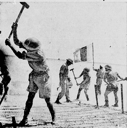
Men of the British Pioneer Corps are literally paving the way for further advances in Sicily. They swing their mallets hurriedly as they make a wire road along the beach.
