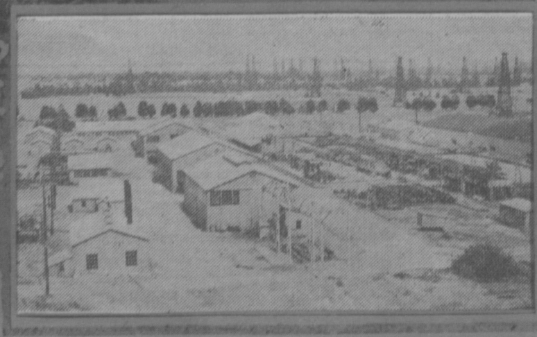
VIEW OF C.C.M.O. SHOPS AT TORRANCE
