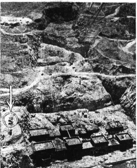
From top of cableway head lower, 700 feet above Sacramento River, this is way embryo Shasta Dam looks after 40,000 cubic yards of concrete have been poured. Six million cubic yards will be poured, under supervision of U. S. Bureau of Reclamation, in 50-foot square blocks which are raised in alternate rows in successive five-foot lifts. There are five trucks in arrow-marked circle at left, incidentally.
