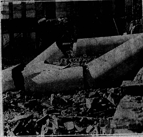
It may be earthquake weather in Southern California, but the picture above is not that of damage done by a temblor. The stately Greelan columns of the Van Nuys, Cal., High School are shown just after their final destruction to make way for a more modern, earthquake proof, building.
