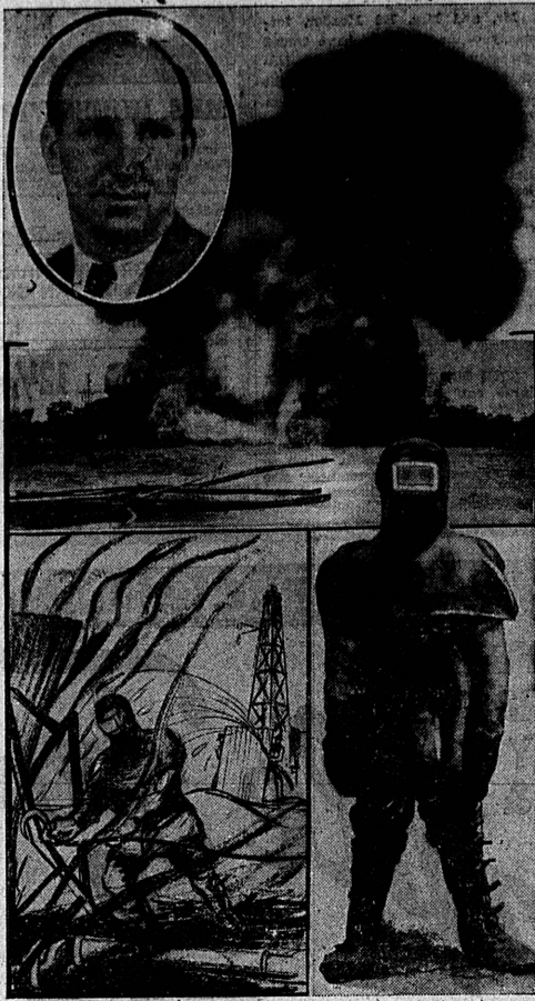
Fighting the danger of the oil field—once the fire zone is clear of metal... A photograph of M. M. Kinley of Tulsa, expert, who has put out more than 60 blazing wells in his asbestos suit which he goes to battle. To the left is shown how Kinley goes into the flames, while his assistants play a wicket on him, to remove iron rigging, tools, etc., which must be taken clear of the blaze before he can "shoot out" the flame with nitro-glycerine.
